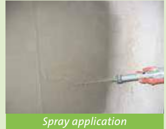
Large surface restoration
