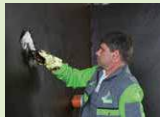
Waterproofing against Radon
