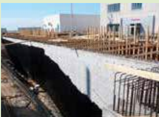
External basement waterproofing
