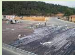
Floor slab waterproofing
