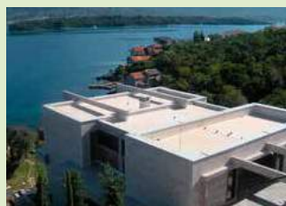
Liquid roof waterproofing
