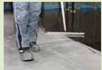
Coating after 24 hrs
