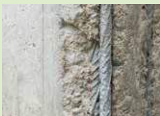
Corrosion protection (coating)
