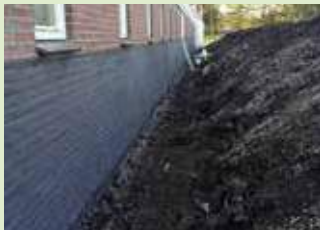
External basement waterproofing
