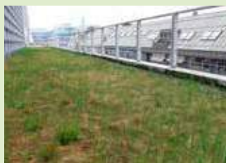
Under ballast / green roofs
