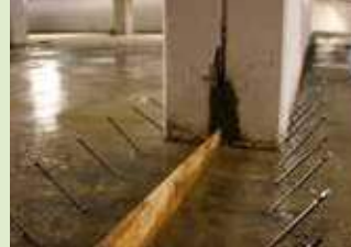
Water-bearing joints
