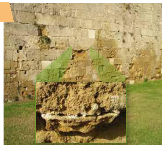
Salt crystals on the surface
