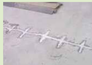
Crack stitching
