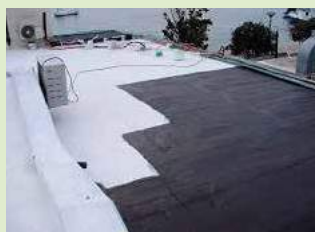
Waterproofing on bitumen
