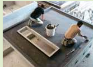
Precast concrete production
