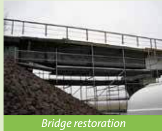
Restoration of support beams
