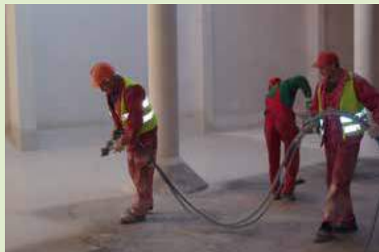
Drinking water tank, Tarnów, Poland
