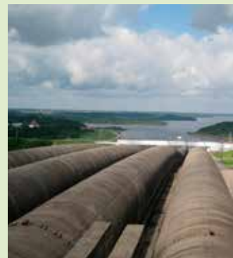
Water power plant, Lithuania
